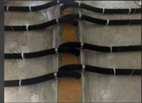
Flexible tubes move with the liner and distribute up to 1/7 CFM/bu of air from the center trough through the grain.
